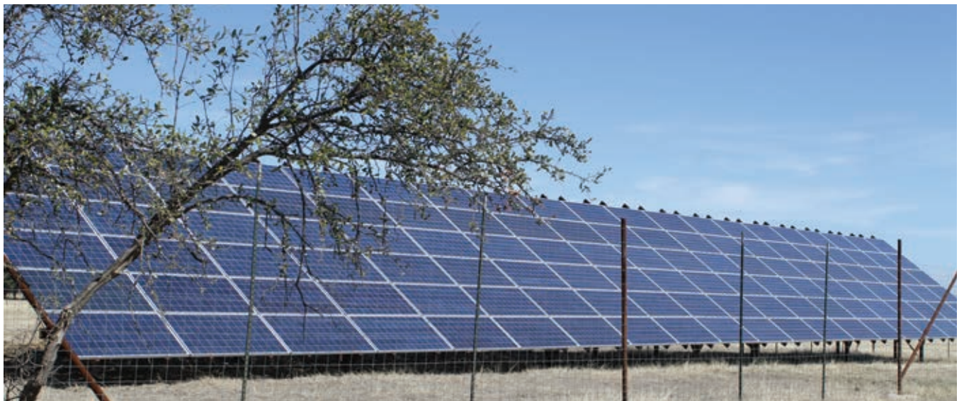
The ranch's solar array is a 37-kilowatt unit capable of producing 73,112 kilowatt-hours annually, enough to power five average-sized homes.
