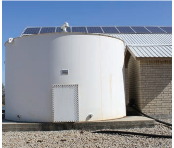
The guest house features a 7-kilowatt solar array and a 3,200-gallon water cistern. However, with no backup battery storage, this location does not possess self-sustaining capabilities.
