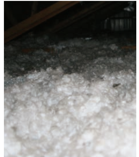
Fluffy mounds of blown-in insulation help cut heating and cooling costs.
