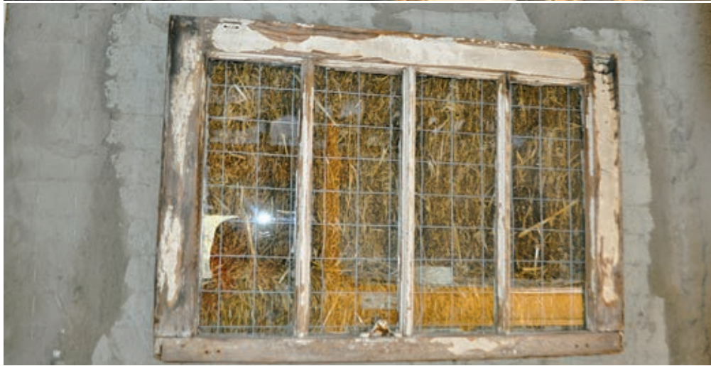
TOP: It was Laura's job to stucco both the inside and outside of the home. Laura said the stucco was the most time-consuming and difficult job of the entire project. 'I built up some pretty good muscles doing the stucco,' she said. MIDDLE: The stucco is applied, and once the house is painted, it will look much like any other conventional home. BOTTOM: Inside the house, beside the living room door, Creath and Laura installed a 'truth window.' After the home is completed, visitors will be able to see inside the walls and observe how the home is constructed using the bales.
