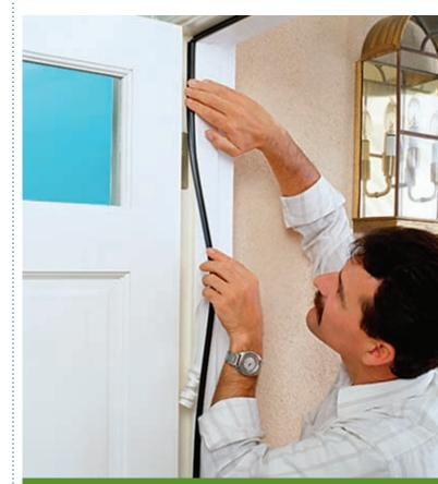
Weatherstripping around doors is an inexpensive and easy way to save energy.
